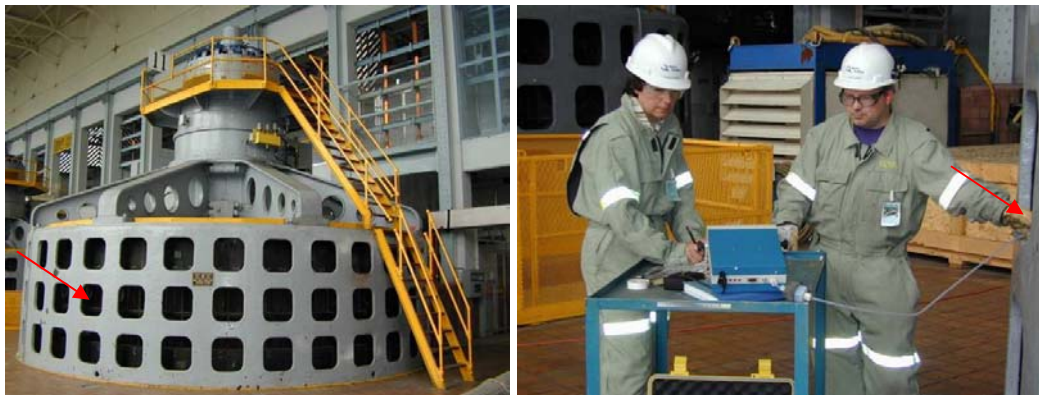
Example of sampling ozone from the cooling air exhaust of a generator. Arrows show a typical monitoring position.
